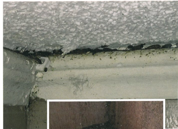
Above, crown molding made ideal harborage for the German cockroaches. Right, feces, cast skins and debris made the house uninhabitable.
